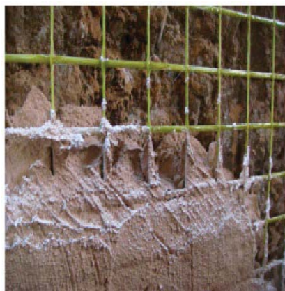
Fig. 2. GFRP application to the masonry wall.
