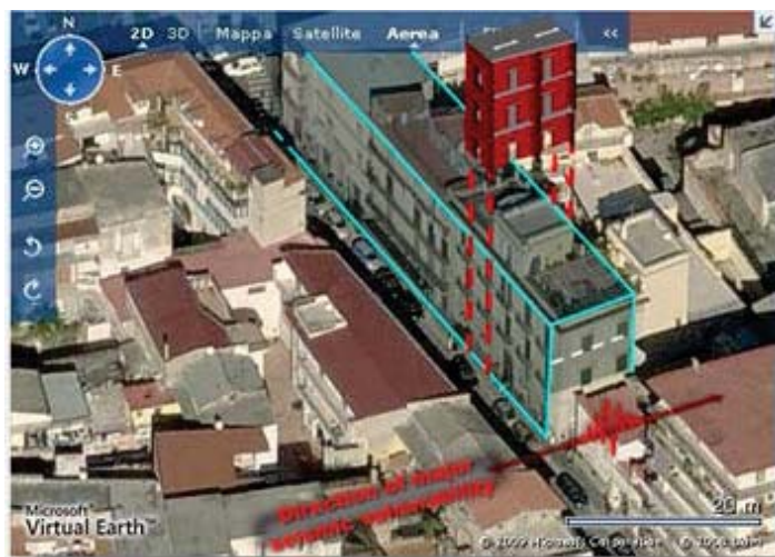
Figure 1. The case study of a masonry building subjected to a vertical addition intervention.
